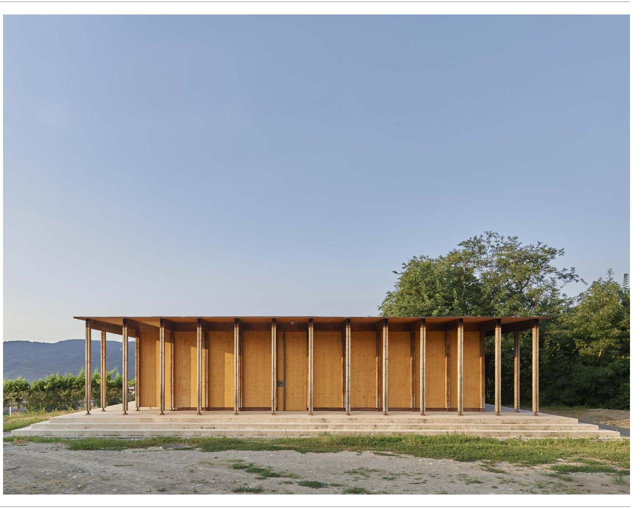
The pavilion consists of a prefabricated fir wood structure. The pillars have a section of  $14 \times 14$  cm. Two of the sides of the pillar are marked by a 2 cm groove. The pillars support 13 laminated fir beams measuring  $794 \times 39 \times 14$  cm made by a local sawmill. The structural parts have burned and brushed finish. The curtain walls are made with yellow construction site panels.
