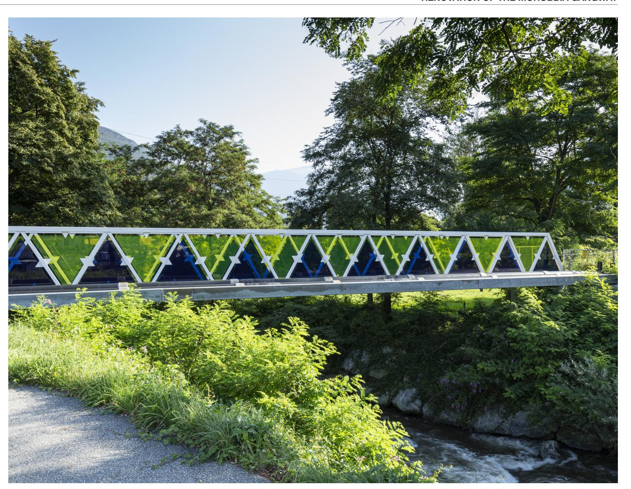
The free space left between the existing structure and the glass pannels allows air circulation, avoiding overheating of the air inside the walkway; the free space between the glass and the structure also guarantees the passage of the wind, reducing its lateral thrust on the structure.
