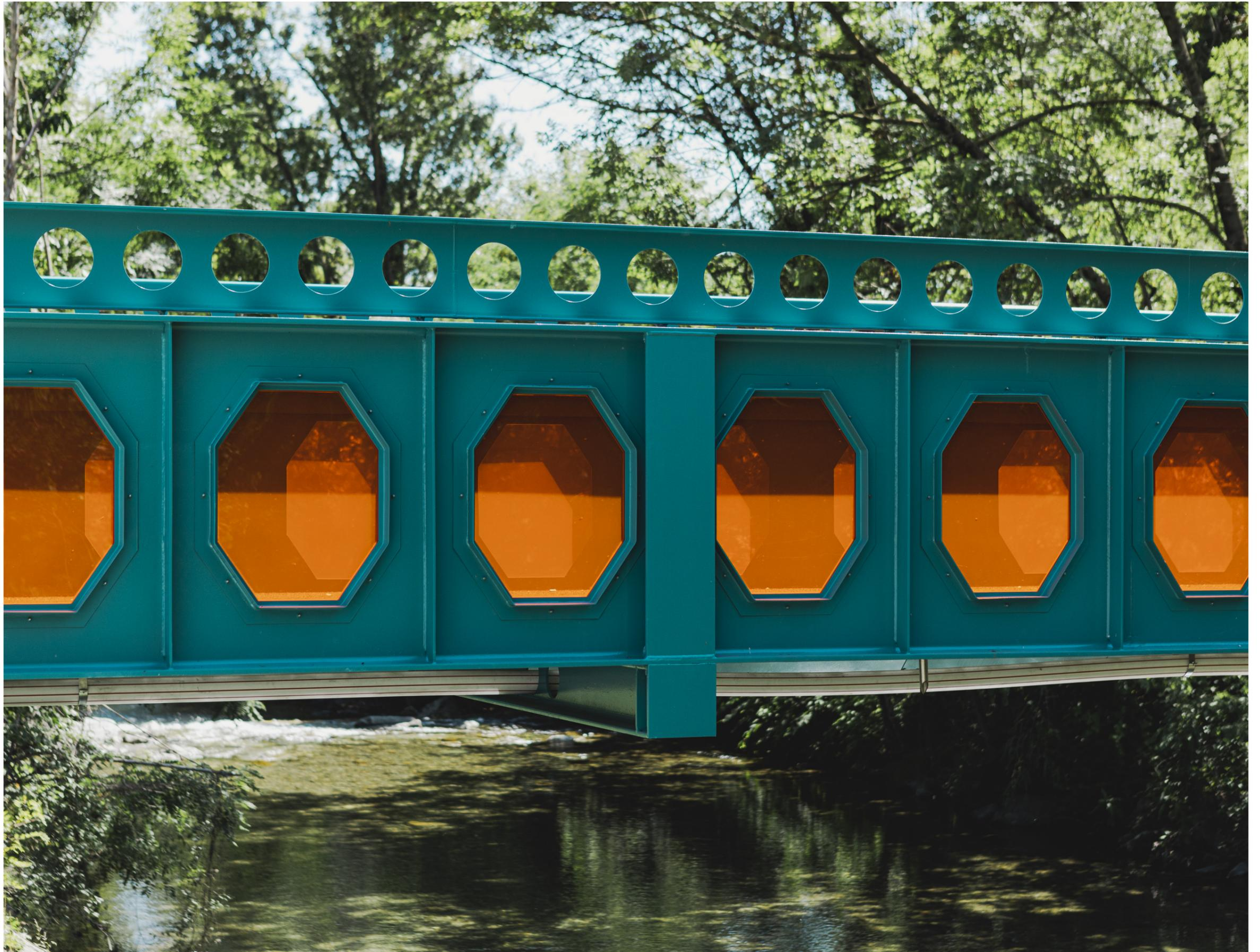
the octagonal holes, special glazing beads have been built. Those fixed to the internal sides of the bridge are flush with the core of the beam, while those on the outside have a 5 cm protrusion which forms a sort of frame that emphasizes the characteristic shape of the hole.
