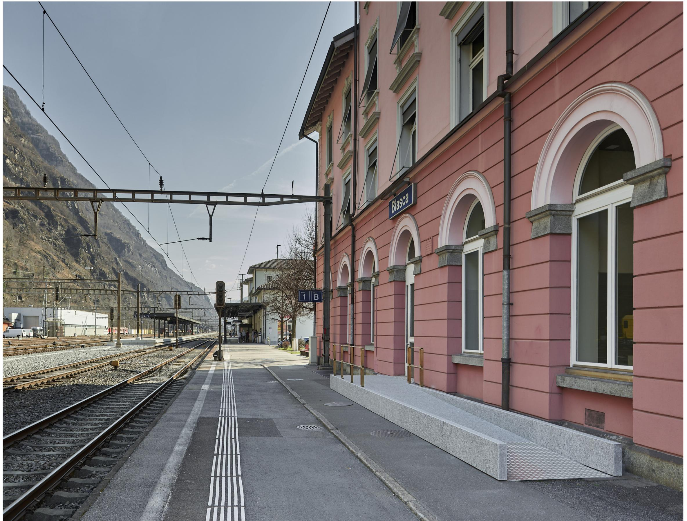
granite slabs for the footing and 10 cm for the side infill.
